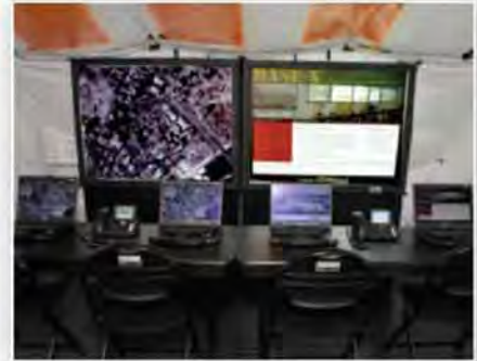
4 Man Command and Control Center
